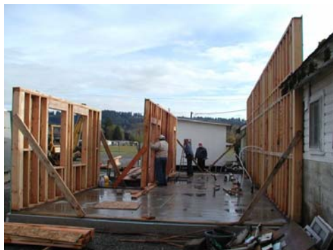
Lab walls going up for SOD lab
